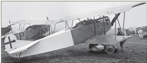
This unidentified late production Fokker D.VII (Alb), possibly from Jasta 18, was photographed in American hands after the armistice. Note the fully louvered engine side cowls (K19 & K23). The style of the additional cooling hole cut into the top cowling under the high exhaust and the white and red(?) fuselage are consistent with aircraft from Jasta 18. A late production OAW built Fokker D.VII "P" can be seen immediately behind.
