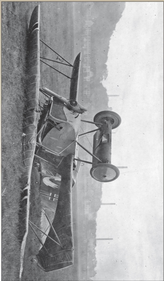
This is a very rare photo showing a 160hp Diamler-Mercedes D.III engine fitted into an unidentified Albatros built MEJ Fokker D.VII. Although almost certainly featuring internal upgrades to boost performance it is very unusual to see this type of engine powering a Fokker D.VII, which gives some insight into the engine supply problems facing the Germans towards the end of the war. Note the small vertical air pump (55) , springs centered on the rocker boxes (56) and high exhaust (57) & (58) details. The nose cowlings appear to have received a coat of yellow paint and there is a comet marking painted on the side of the fuselage.
