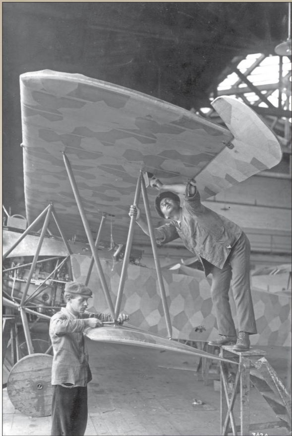
An Albatros built Fokker D.VII nears the end of assembly, presumably at the Albatros Johannisthal factory. Note that the fuselage and top wing are covered in 4 colour lozenge but the aileron has 5 colour fabric applied. The wooden wheels are temporary installations for moving about the factory.
